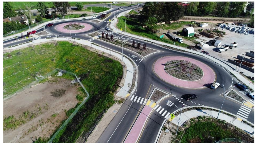
SR-198 and Farmersville Blvd Roundabouts (Farmersville, CA)
