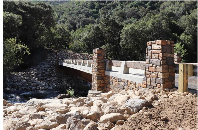
Mineral King Road over S. Fork Kaweah River Bridge (Three Rivers, CA)
